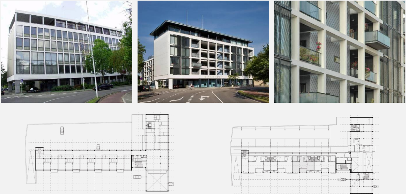
Figure 3: Granida. Left: the building before conversion; right: the building after conversion. The location near the city centre and the image of the building were important success-factors for this conversion. Alterations of the façade and a bad technical state of the structure led to high construction costs.
